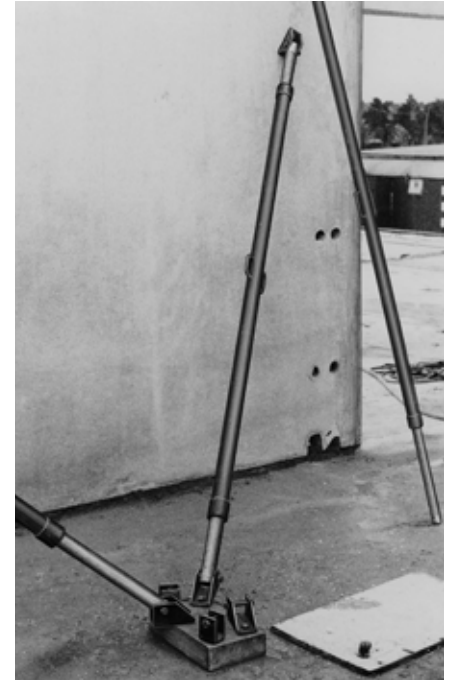
3-dimensional swivel-end accommodates any slope or angle with single bolt fix
