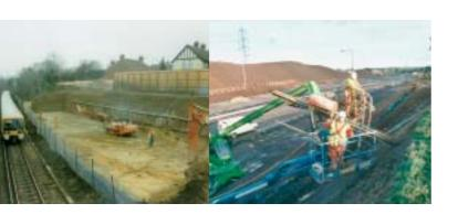
Soil nailing is an efficient, effective and economical method of earth reinforcement, which allows a controlled improvement of the natural stability of the soil.
