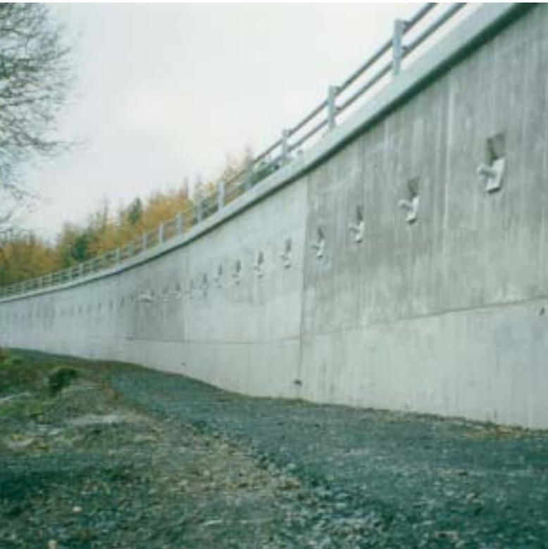
Ischebeck Titan Anchor Piles can be used wherever a traditional ground anchor is being considered and provide a rapid, efficient method of installing tie back anchors in one visit to the drill hole.
