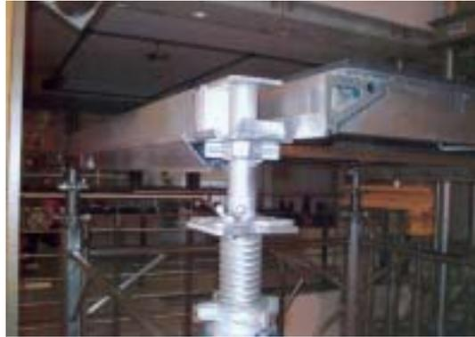
Drop-head allows quick release of all primary beam and panel components for re-use, maximising productivity and utilisation.
