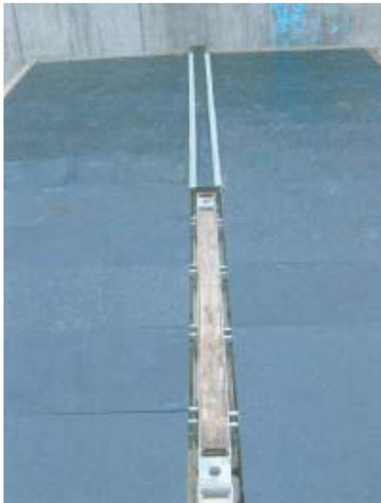
Hard-wearing GRP synthetic faced panel and in-fill strip give high quality finish.
