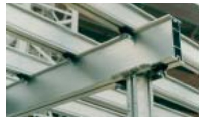
Headplate to beam fixing
