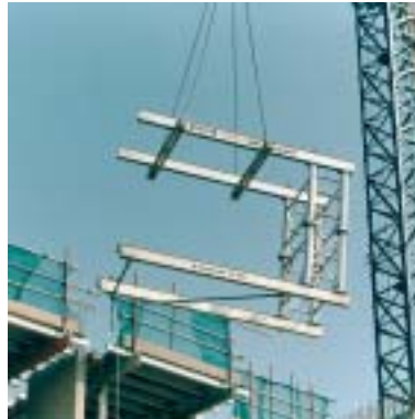
'C' hook For removal of small edge tables.
