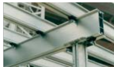
Headplate to beam fixing
