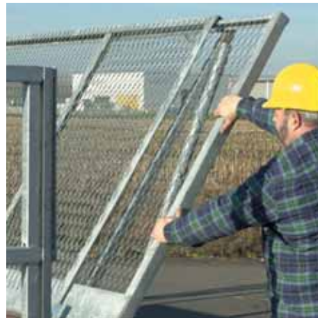
Protective grille extension.
