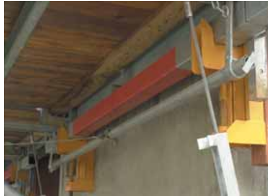
Support beam and locking device secure platform to structure.
